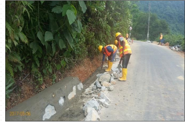
L Drain Construction @ Ginigathhena Dehigasthenna Ella Uda Road, Road No- 46 CH 2+930 – 2+940
