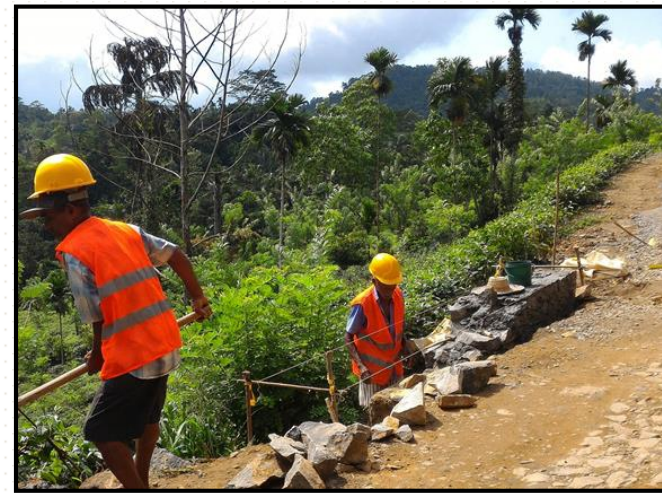
Head wall minor repair Halwitigala Janapadaya - Tawalama Mukalana Road CH 01+235
