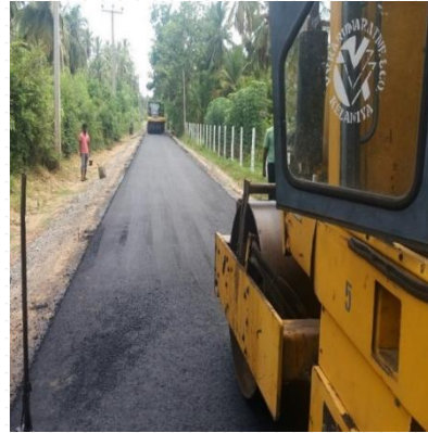
Asphalt Compaction at Road ID 26 0+700 - 0+800 km
