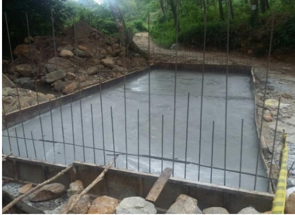
Causeway encasement base concreting at Hallina junction to Polwattahena Matihakwela Hunuwala Road, Rd No.3 Ch.5+420 RHS
