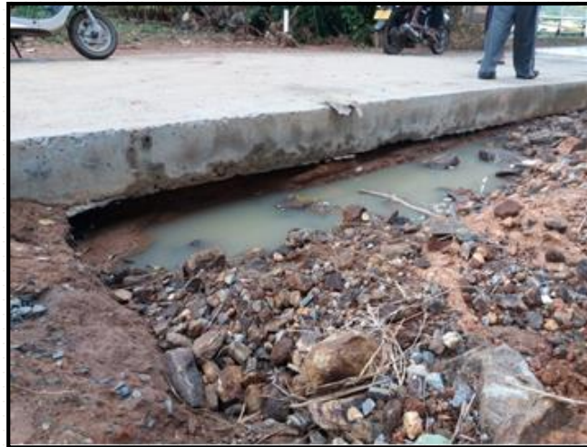
Shoulders Damaged; Agulmaduwa-Aranwela Road CH 1+240(RHS)
