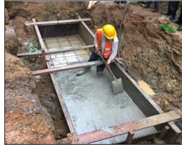
Culvert Head Wall Base @ Road No 63 Ambepussa Dadli Senanayake Rd CH 1+824
