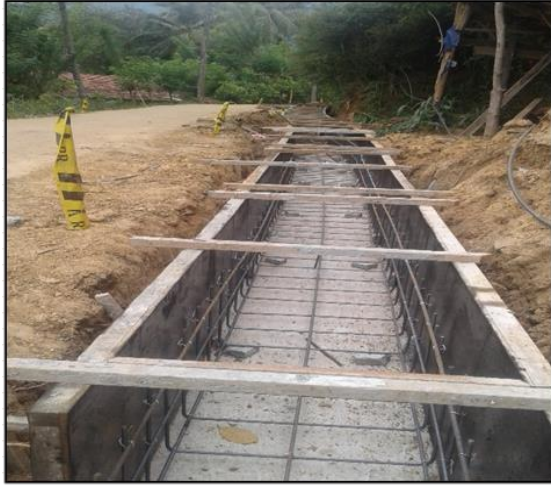
Construction of retaining wall at Ch.(1+530~1+580)km at Thapaswara kanda road (Road ID 08)
