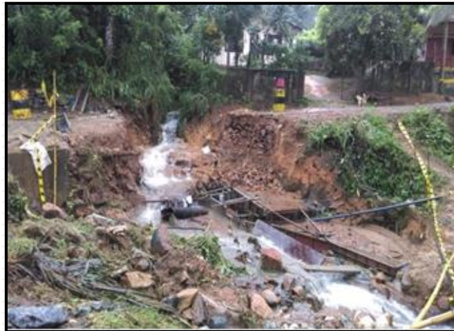
Shuttering & Formwork Damage; Pangirihena – Mayakaduwa Road, CH 01+498
