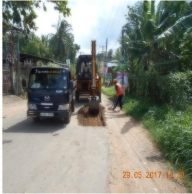
Excavation for Edge Widening at Road ID 71 4+120 km
