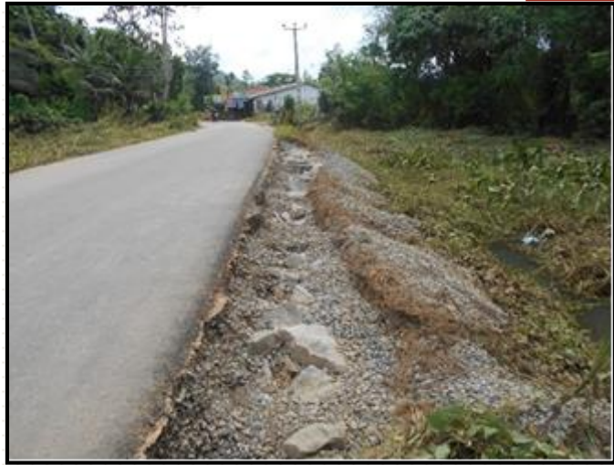
Shoulder Eroded; Akuressa – Katanavila Road (ID 4), CH 03+150 - 03+230 (RHS)
