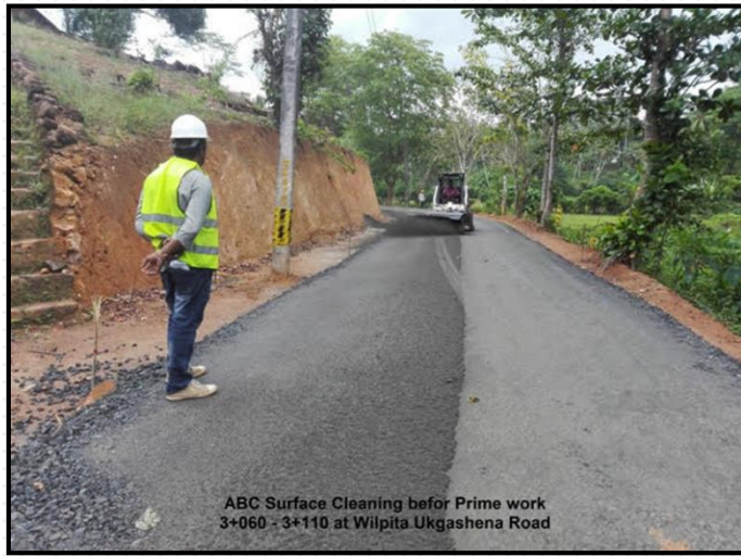
ABC Surface Cleaning Wilpita Ukgashena Road, CH 03+060 -03+110
