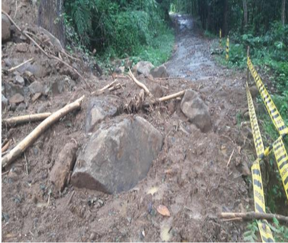
Earth slip at KaluAndura Diurumpitiya watta - Gatahaththa Road via Muruthengala, RD 17 Ch- 01+800
