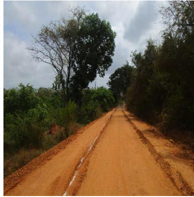
Shoulder Construction at Road ID 08 0+000 - 2+700 km
