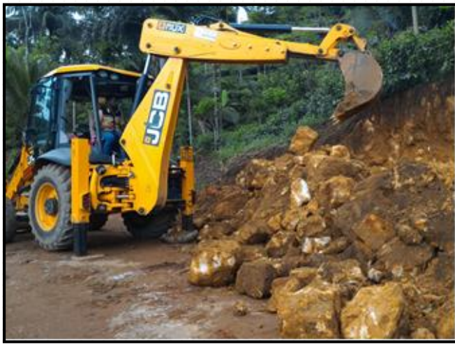
Rock Excavation; Halwitigala Janapadaya - Tawalama Mukalana Road, CH 01+829
