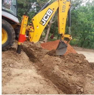
Replacing Existing Water Line at Road ID 92 4+283 km
