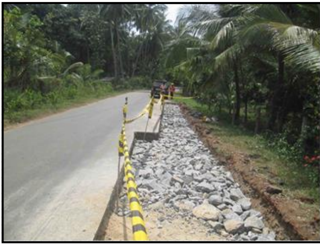
Base failure Construction; Perahara Mawatha/Mulkirigala School Road, CH 01+300
