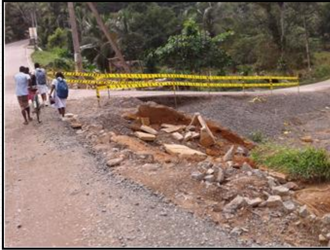
ABC Washed Out & Shoulder Damage; Mavita Duliella Road, CH 00+000
