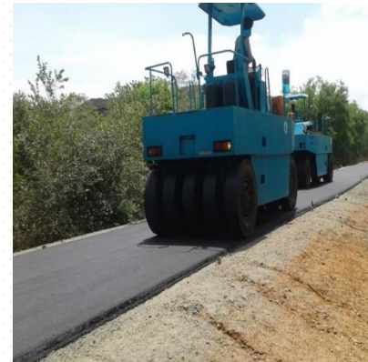
Asphalt Compaction at Road ID 68 0+690 km
