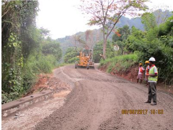
DGAB construction at Ch. 0+710 – Birindiwela - Walawela , Dullewa RN 56
