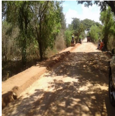
Shoulder Construction at Road ID 57 4+750 km
