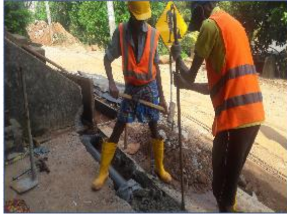
Sewer Line Laying CH 1+830 – 1+845 RHS Viharagama Watadeniya Road (KRN 28) Date 17/05/2017
