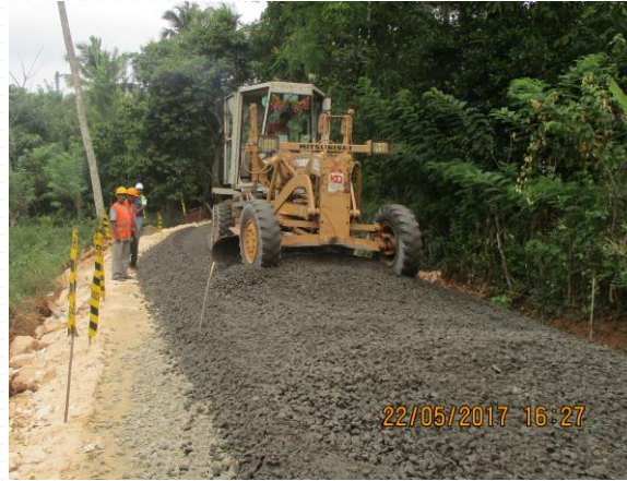
DGAB construction at Ch. 01+450 – RN 02
