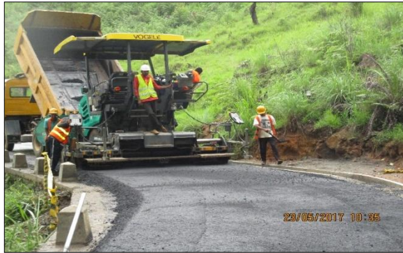
Asphalt paving @ Welioya Shanen Road Road No - 41 CH 7+480 – 7+600
