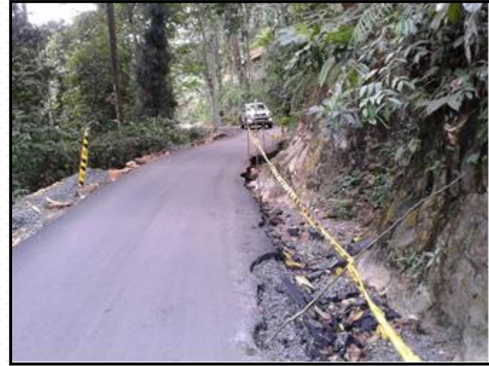
Erroded Shoulder; Udugama - Kothalawala Road.
