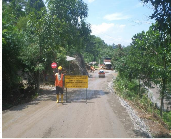
ABC Compaction Work at Galabada Rathgaga temple to Palabaddala Road via Kudawa & Mapalana, Road ID 13 at 01+250 Km on 05.05.2017
