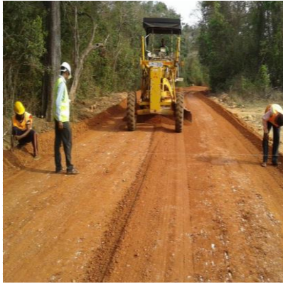
Sub Base laying at Road ID 33 3+220 - 3+310 km
