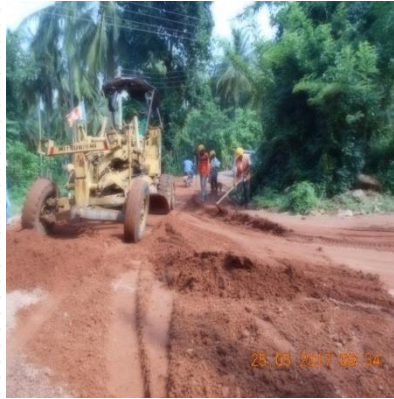
Sub Base Laying at Road ID 38 4+225 km
