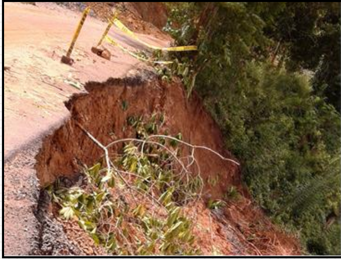
Asphalt and Shoulder Damage; Deniyaya - Viharahena Road (24A).
