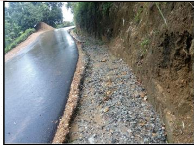
Asphalt & Shoulder Damage; Janahitha Tea factory - Muslim Janapadaya Road, CH 00+450 (RHS)
