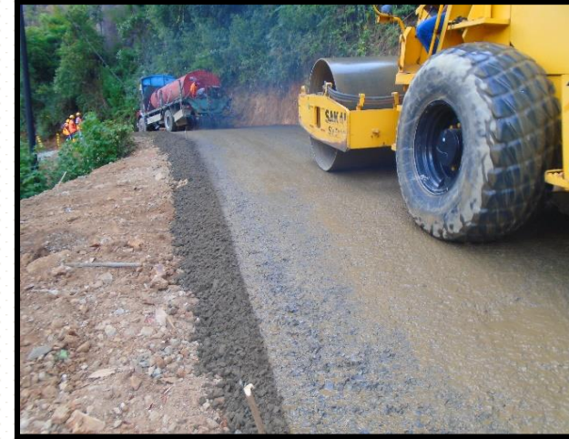
ABC compaction @ Ragala Starapet Panditha Kumburakotambe Road Road No - 03 CH. 5+530-5+630
