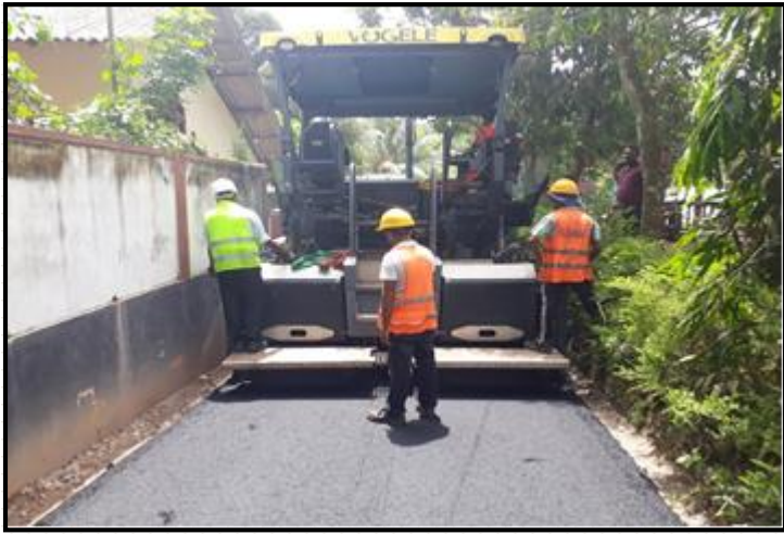
Asphalt Laying; Poorwarama Bataduwa Road, CH 01+100
