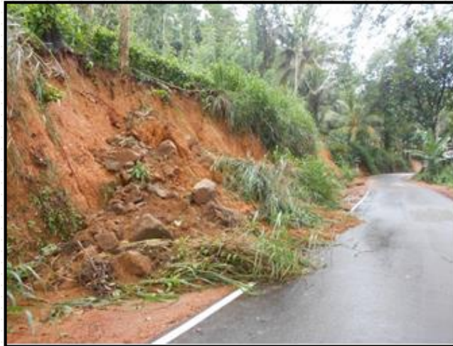
Earth Collapsed; Urubokka – Pothdeniya Road (ID 42), CH 05+570-05+580 (RHS)
