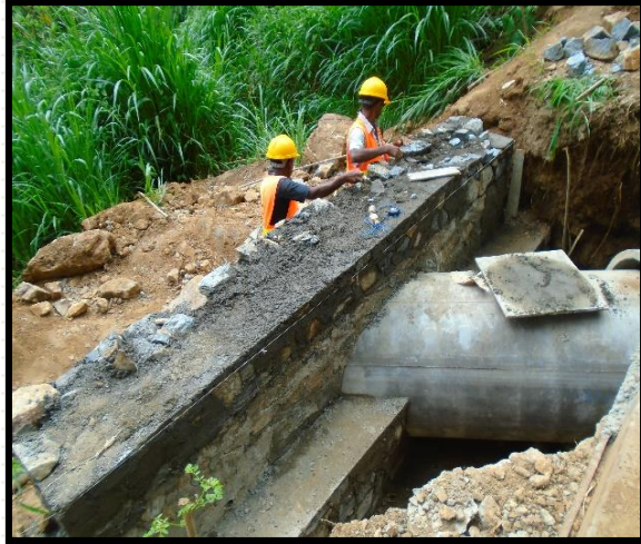
L drain construction @Mahauva - Highforest Road Road No – 10 CH 1+330-1+360
