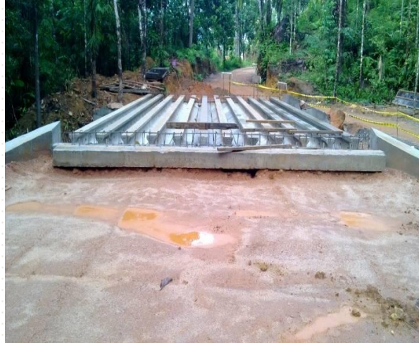
Concreting deck slab of bridge at Ch.0+286 km in Thapaswarakanda road (Road ID 08)
