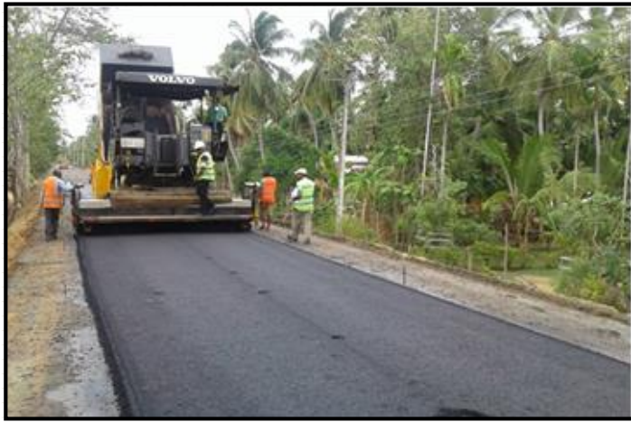
Asphalt Construction; Siyabalapahena Road, CH 00+820
