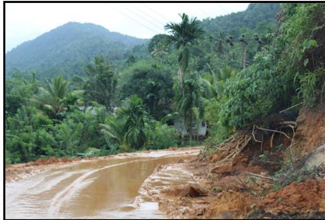
ABC Washed Out & Shoulder Damage; Mavita Duliella Road, CH 00+000
