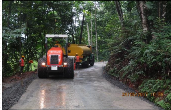
DGAB Leveling & Final cutting @ Pallewatta Dagampitiya Notan Road Road No – 47 CH 5+656 -5+676
