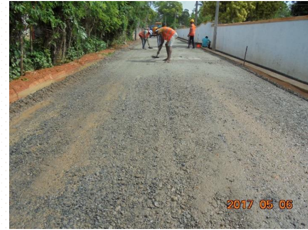
Surface Preparation at Kurudippita Road, Road ID 35 Ch. 0+380 -
