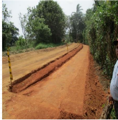
Embankment Construction at Road ID 10 1+400 km
