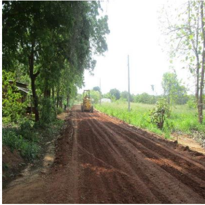
Sub base Construction at Road ID 43 5+500 km
