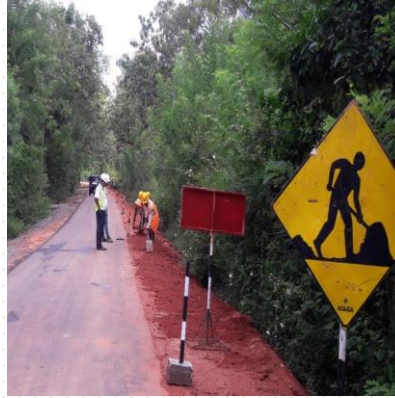
Shoulder Construction at Road ID 45 2+300 km
