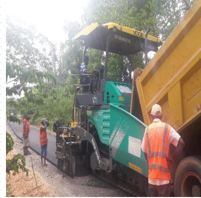
Asphalt Laying at Road ID 92 2+620 - 2+700 km
