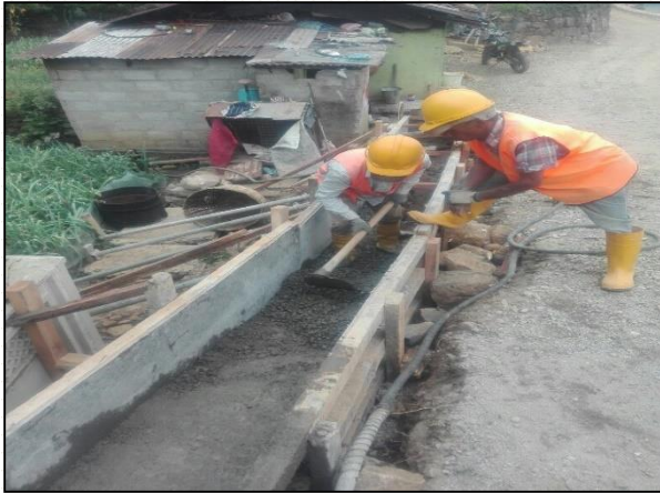
Formwork for key concrete @ Nanuoya - Udaradalla Road Road No-29 CH 5+022- 5+030
