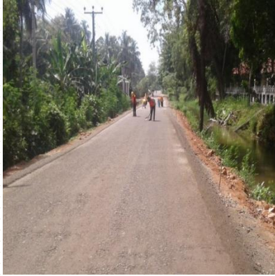
Preparation for Priming at Road ID 25 2+050 km
