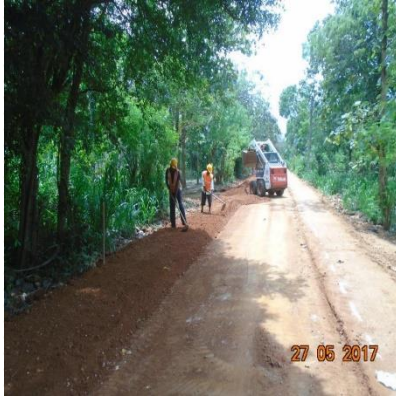
Shoulder Construction at Road ID 28 4+500 km
