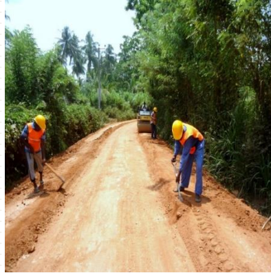
Shoulder Construction at Road ID 48 0+090 km
