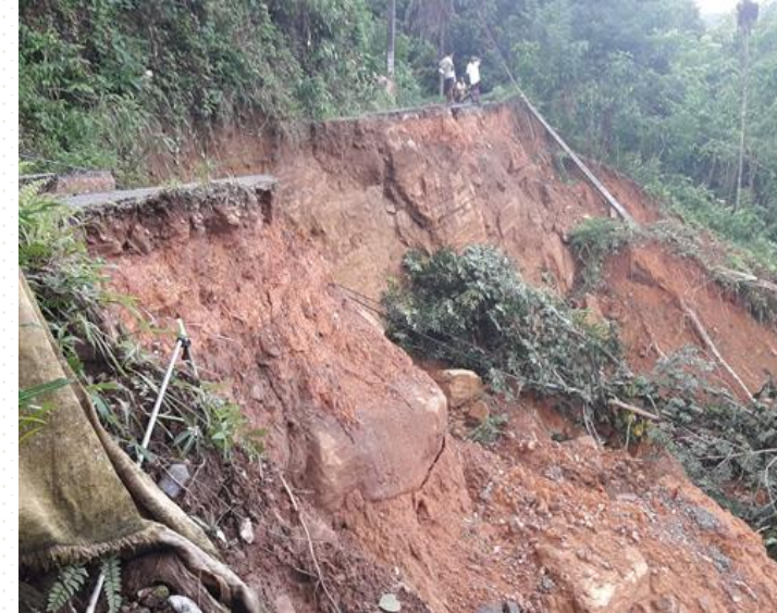
Earth Slip at Polegoda Ihala Welgama Paragoda via Wadigangoda road Road ID 23 Ch-1+600
