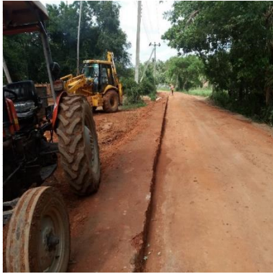
Shoulder construction at Road ID 16 0+700 km
