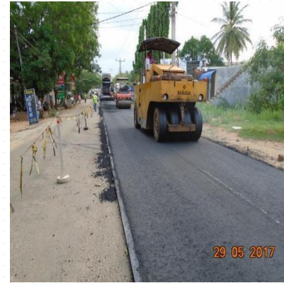
Asphalt Compaction at Road ID 47 0+900 km
