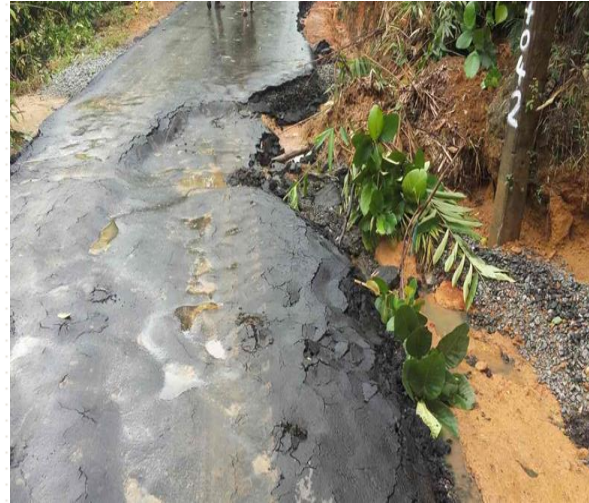
Asphalt surface totally damaged at Elapatha Damme Junction Road (ID 29) at CH 2+042 BS Date 30.05.2017
