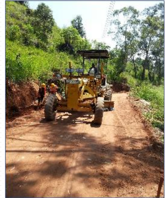
Shoulder Correction work CH:4+950 - 5+030 Manikkawa Junction to Gonadhikawatta Road (KRN 27) Date:02/05/2017
