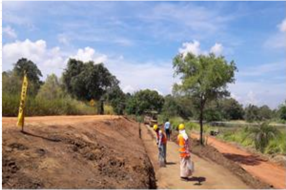
Widening of Tank Bunt at Ch.03+200 – Kandalama Rotawewa Road RN 22
