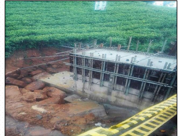
Bridge abutment construction @ Thalawakale - Galkanda Road Road No 23 CH 3+375 LHS
