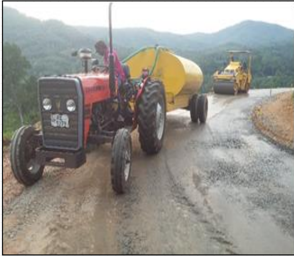
ABC Compaction @ Road No 35 Pindeniya Bridge weliwanguwa Rd. CH 0+570 -0+670
