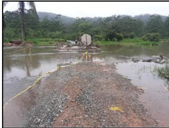
ABC Washed Out & Shoulder Damage; Pinikahana – Puwakdola Road, CH 00+500
