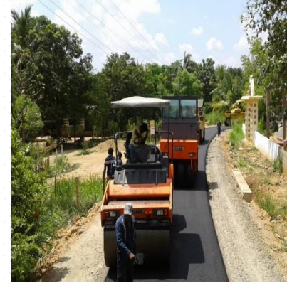
Asphalt Compaction at Road ID 08 1+800 - 2+000 km
