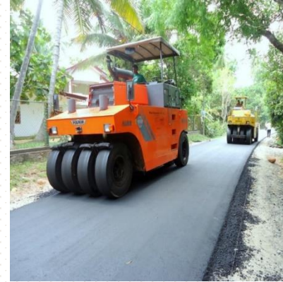
Asphalt Compaction at Road ID 47 8+400 km
