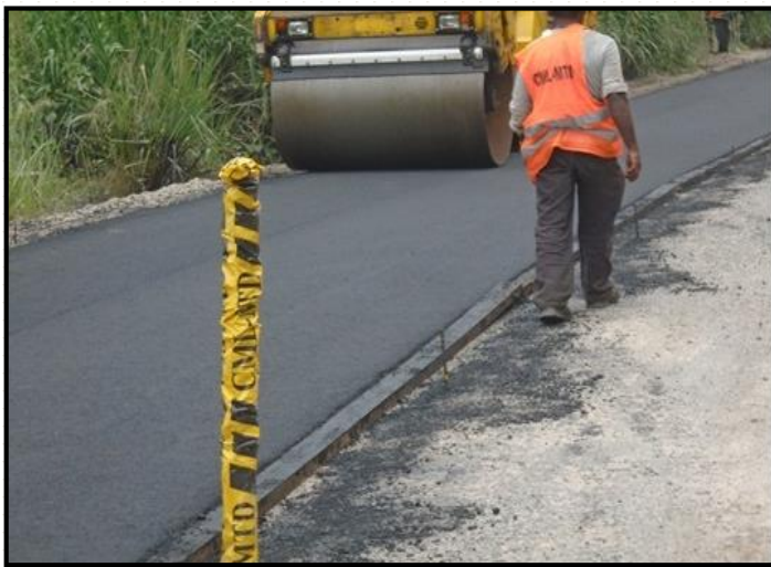
Asphalt Laying; Deniyaya – Viharahena Road, CH 02+410 (RHS)
