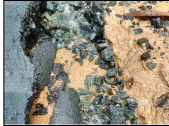
Asphalt Damaged; Sumihirigama Co-op Kakulamandiya hena Mahamadiththa Road CH 0+820- 0+960
