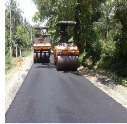
Asphalt Compaction at Road ID 25 1+897 - 2+376 km
