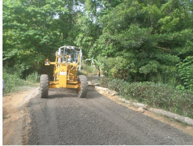
ABC Laying Construction Work at Kuruwita - Kendalanda Road via Eratna (From Kuruwita to Diyarwood Tea Factory, Road ID 11B at 02+200Km on 04.05.2017
