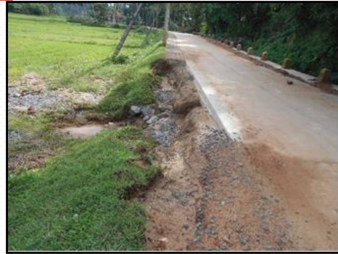
Shoulder Eroded; Abeywuckrama Road, CH 0+630 to 0+640 (RHS)
