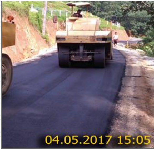
Asphalt laying from 5+540 to 5+570 for Deraniyagala Hospital Road ID-09
