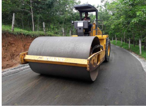
ABC compaction at Kongastanna junction to Ilukkumbura Road, Rd No.5 Ch.2+080- 2+150
