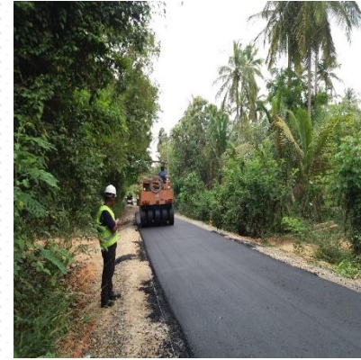
Asphalt Compaction at Road ID 61 0+850 km
