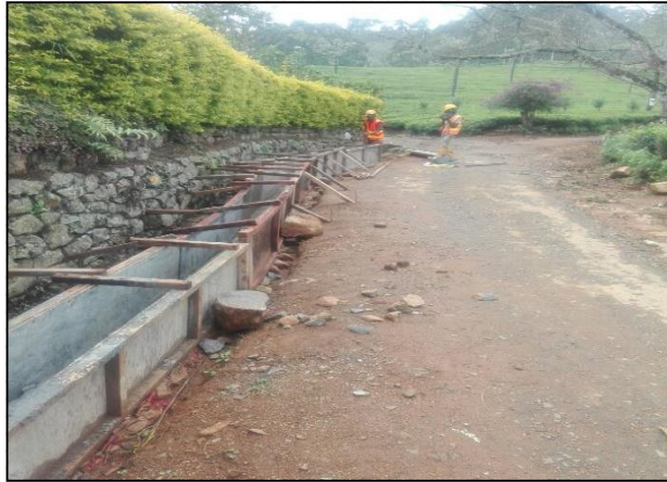
Key concrete formwork @ Rahanwatta - Maussaella Road, Road No 24 CH 2+912-2+928
