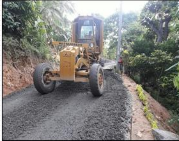
ABC Laying Work at Iskolamuduna junction – Hiloya Road(Watagala Road) via Poddalgoda Road. Road No.4A
