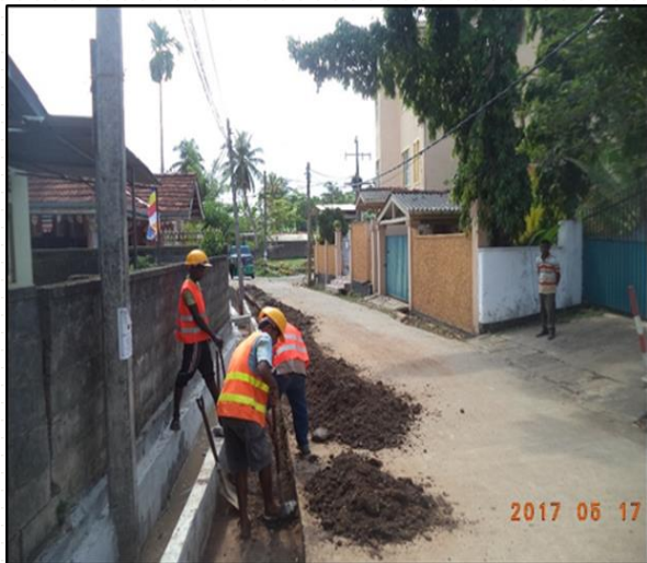
Edge Widening Works @ Solamon Road No 75 0+850
