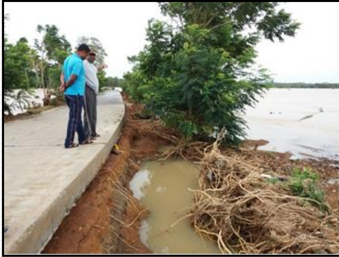
Shoulders damaged; Agulmaduwa-Aranwela Road CH 1+260-1+820
