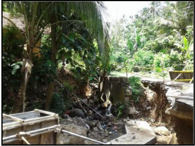
Damaged Culvert; Perahara Mawatha, CH 03+200
