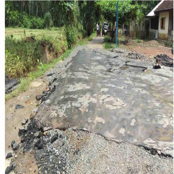
Asphalt surface totally damaged at Elapatha Damme Junction Road (ID 29) at CH 2+900-2+920 BS Date - 30.05.2017
