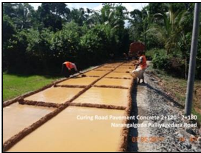
Curing Road Pavement Concrete; Narangalgoda Palliyagedara Road CH 02+120 – 02+180
